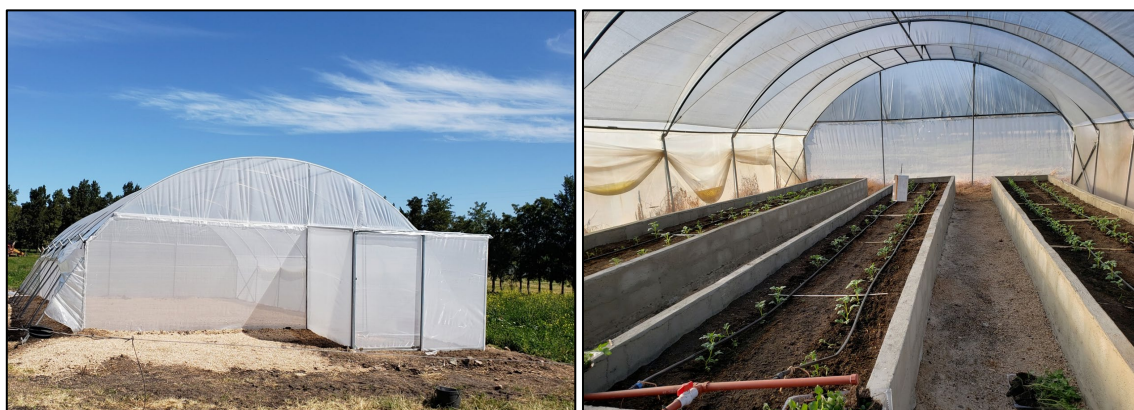
Figure S1: Representative photographs of the high tunnel. Its structure fulfills biosafety level II regulations for GMOs plants. It includes anti-insect mesh, and three replicates (blocks) filled with an enriched soil substrate, contained in elevated cement seed beds, and a disinfection area to prevent outside bacterial dissemination.
